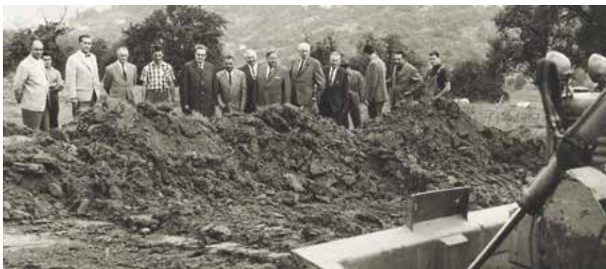
Links: Spatenstich Salzert
